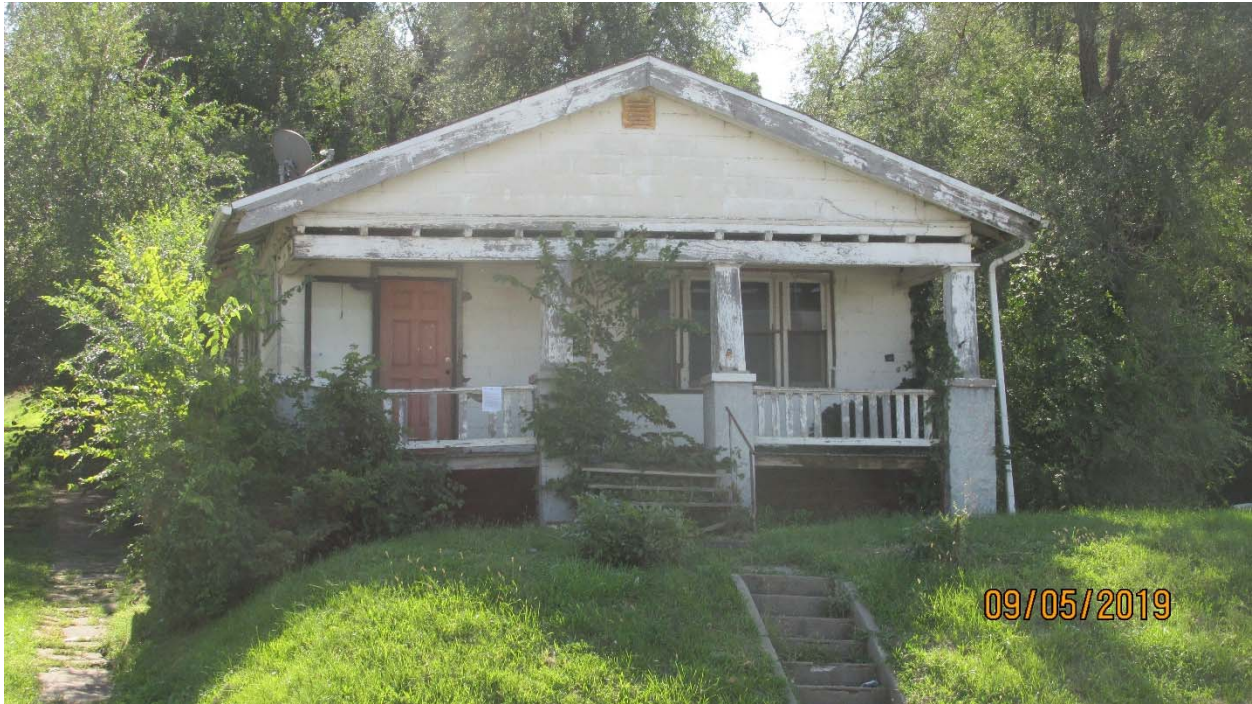
Demolition of 3801 King Hill Ave.
