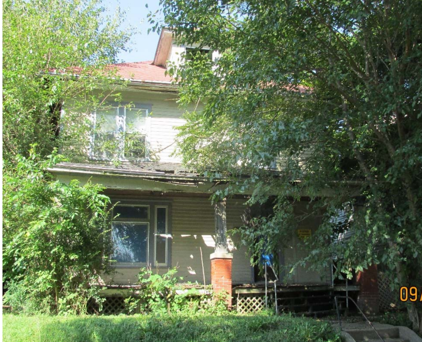
Demolition of 608 S. 15th St.
