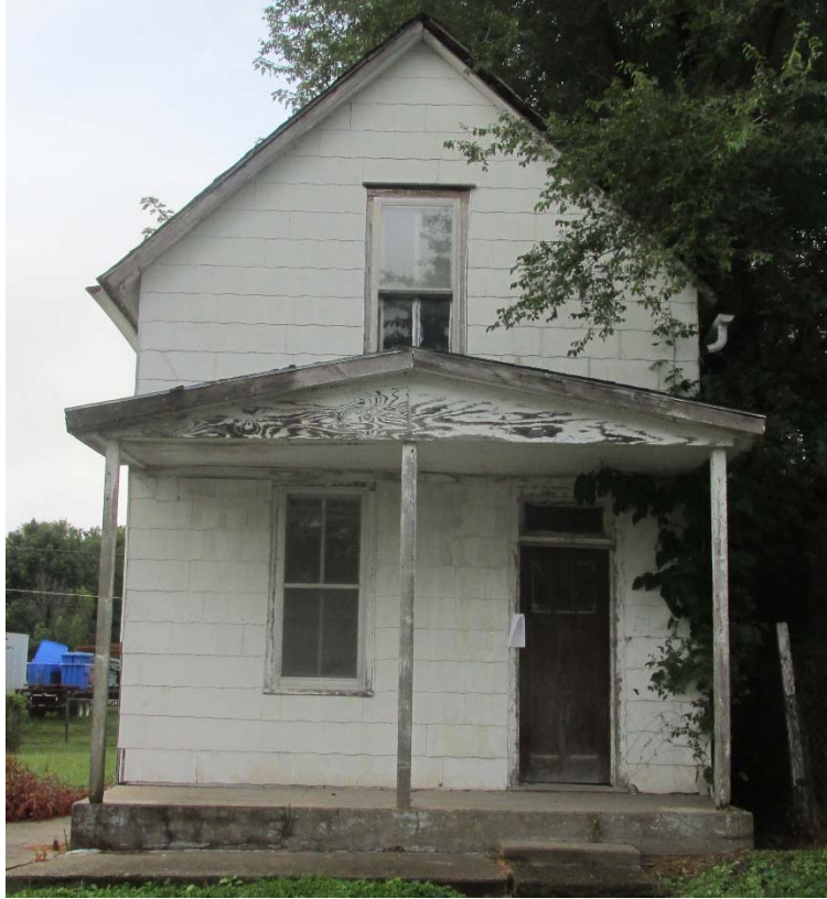
Demolition of 2220 Locust St.
